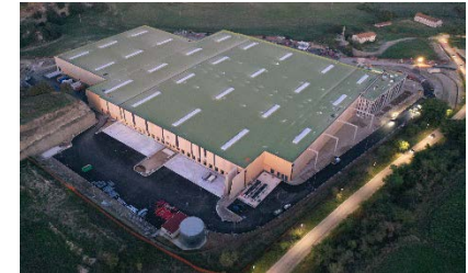
Central-Southern logistic platform (Lazio) works progress
